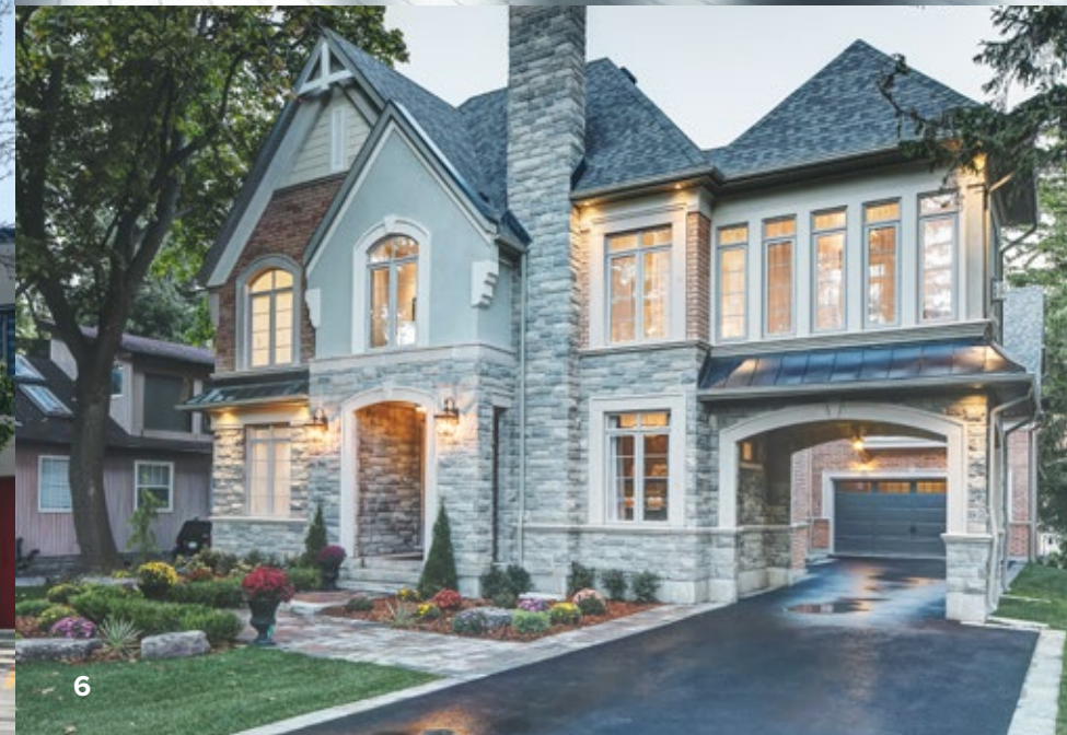
1. 210 SIMCOE, 2. CRAFTHOUSE 3. THE WAY URBAN TOWNS, 4. 400 WELLINGTON WEST (EXTERIOR), 5. 400 WELLINGTON WEST (INTERIOR), 6. FAIRWATER ▲
